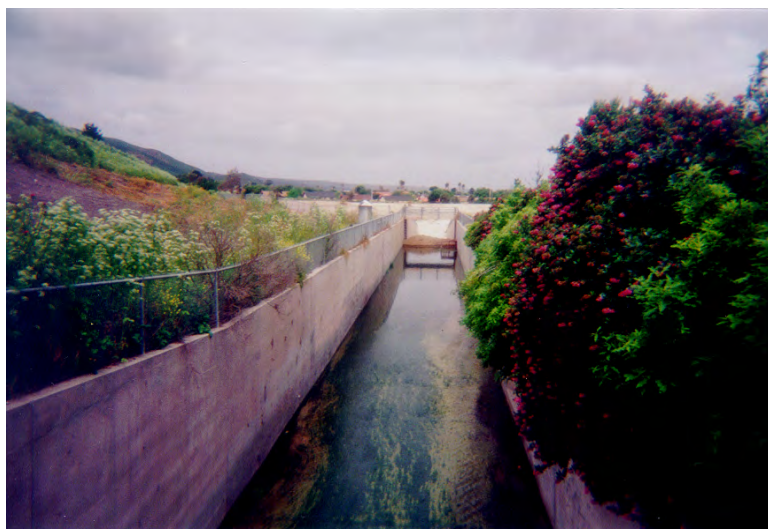
A 3 mile long concrete box culvert confines the lower reaches of San Miguelito Creek
