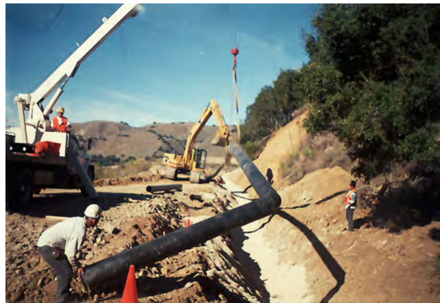
Construction of the Supplemental Watering System Pipeline. Photo courtesy of Barry Longwell.
