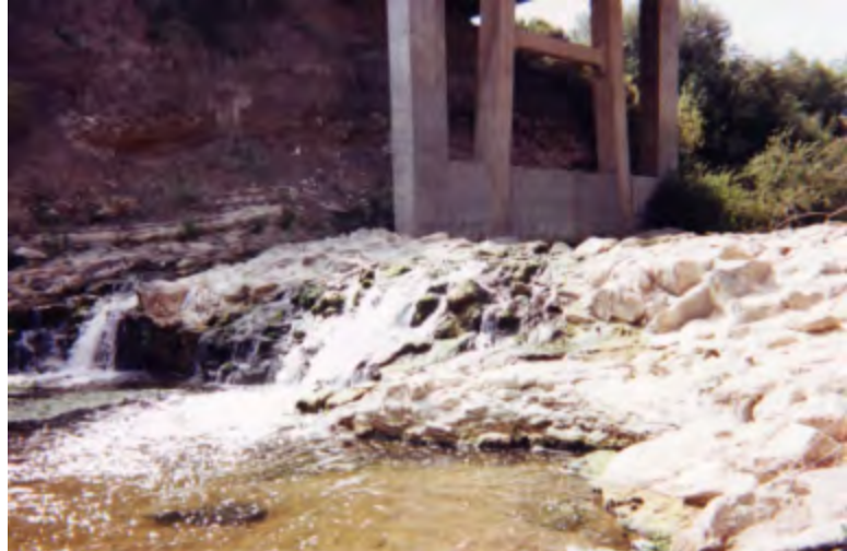
The Highway 1 Bridge apron presents a low flow fish passage impediment on lower Salsipuedes Creek.
